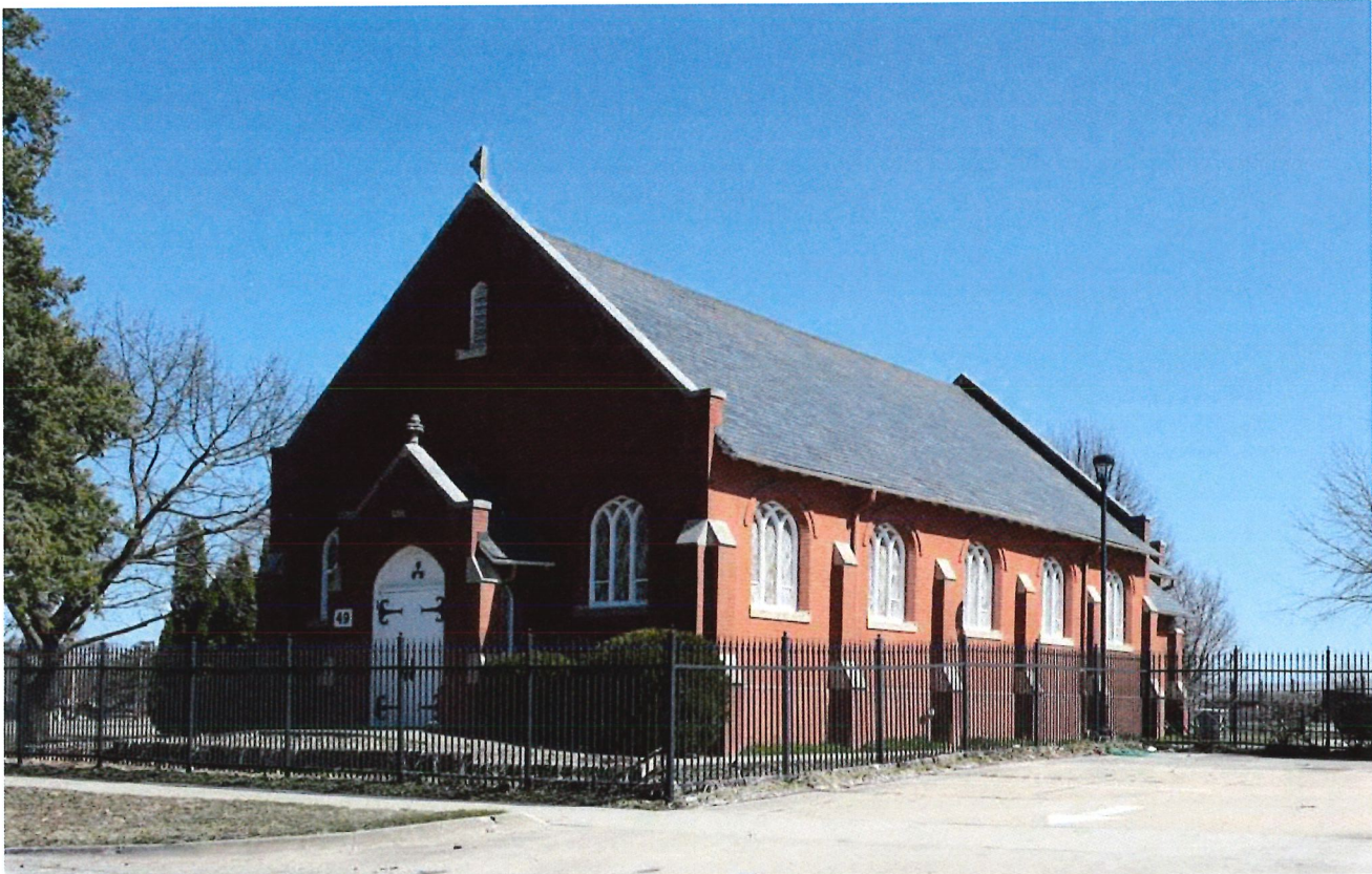
(Chapel exterior, photo by Kelli Lydon)
