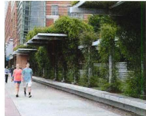
Above: Bridge overpass designs can incorporate vertical screening as was completed at the Atlanta Interstate Bridge.
