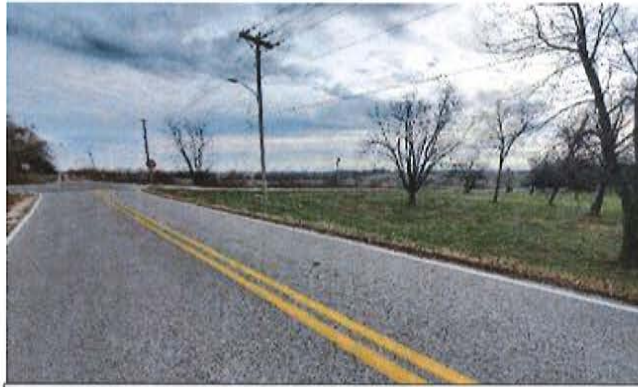
SW McKinley Avenue approaching intersection with SW 56th Street.
