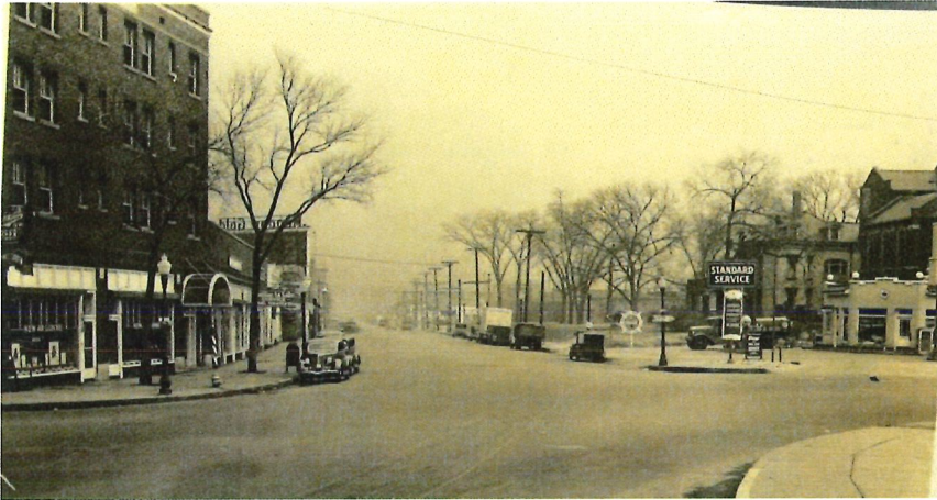
Figure: This 1939 view is taken with the photographer's back to the Ford factory looking east down Grand Avenue, with a rooftop sign for Meadow Gold ice cream visible on the left. This location is about two blocks southwest of the Crescent Chevrolet sign; the Meadow Gold building and sign are now both nonextant. 9
