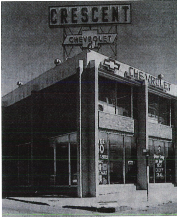
Figure: The Crescent Chevrolet sign was augmented by other signage by the time of this 1996 photograph included in a newspaper special section celebrating the dealership's 65 th anniversary. Additional lighting is visible at the roof edge. 28
