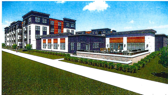
CLUBHOUSE AT PASSEO FROM SOUTH
