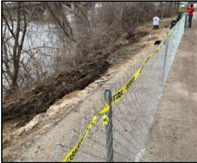
Photo Above: Repair Site
