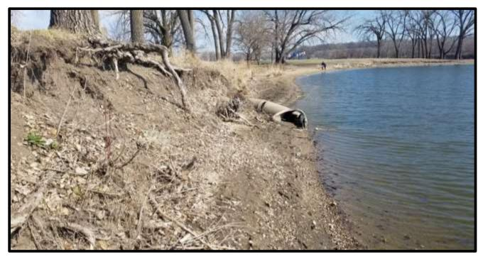
Photo above: North-centrally located 6-foot tall eroded lake shoreline and damaged storm sewer.
