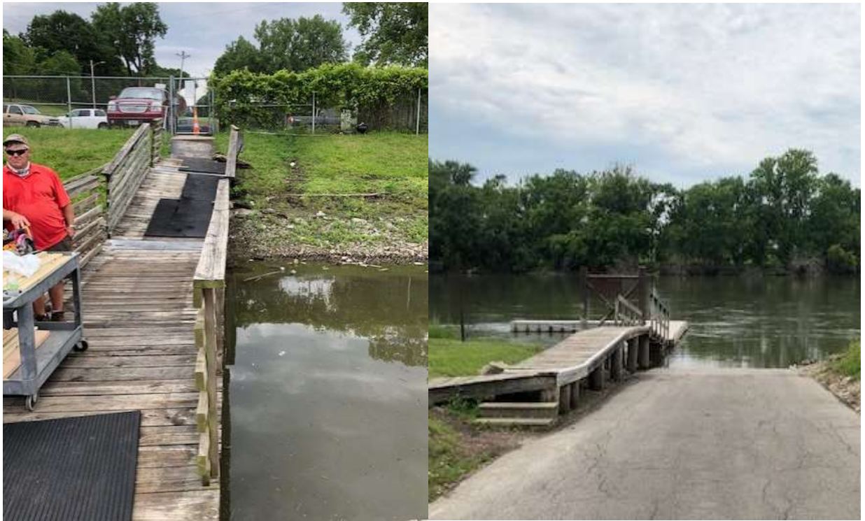
Degraded Streambank and Makeshift Ramp at Captain Roy's
